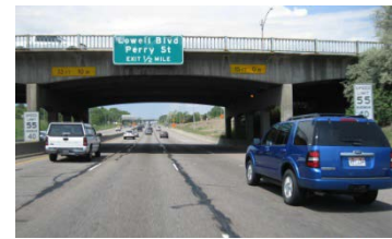
Westbound US 6 at the Federal Boulevard Bridge
