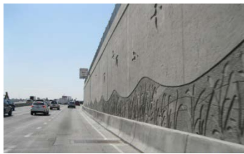
Alameda and I-25 wall treatments
