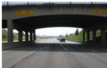
Existing Federal Boulevard Bridge over US 6
