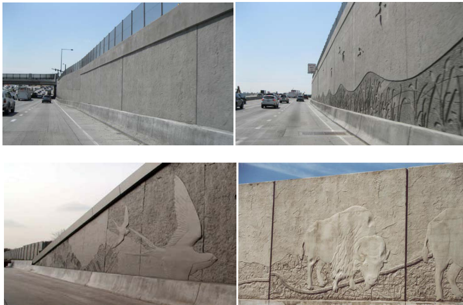
Figure 13: Different Retaining Wall Form Liners and Patterns
